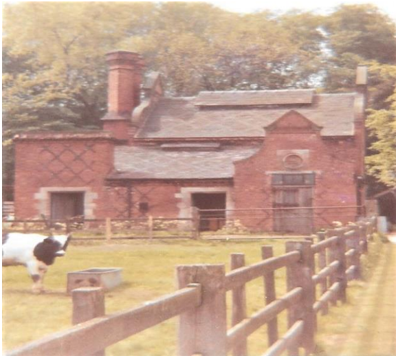
The Old Gasworks
